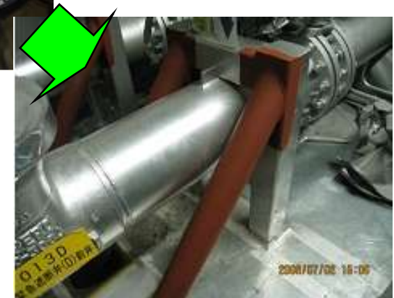
Supports were reinforced and modified into secure structures
