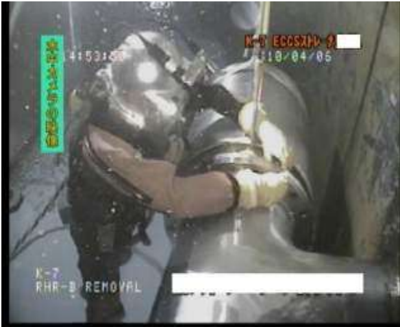
ECCS Suction Strainer (Underwater)
