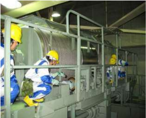
R/B Ceiling Crane
